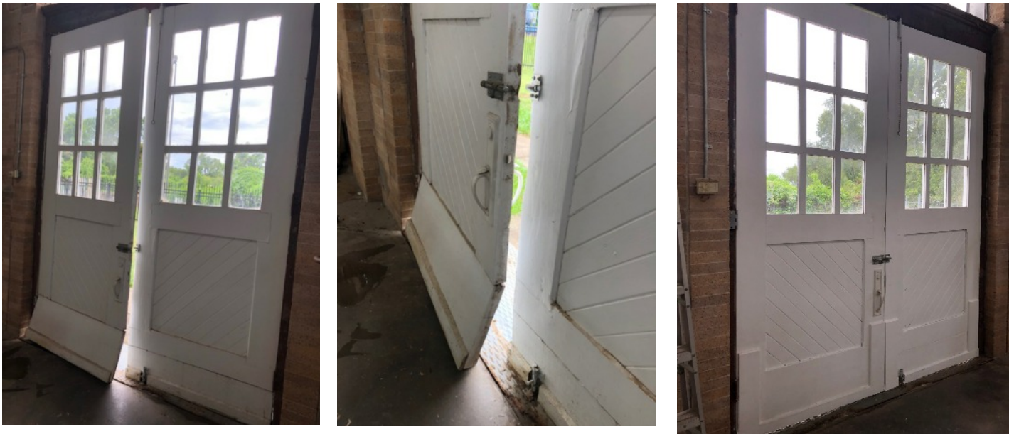
Before and after views of the formerly dilapidated entry doors
