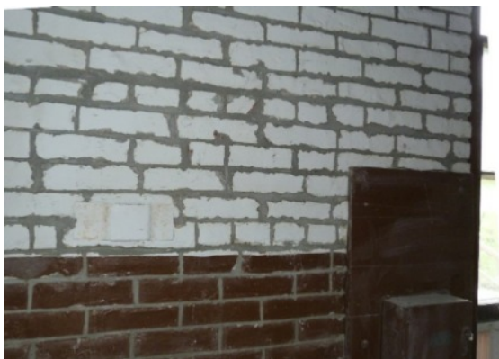
Close-up of repaired wall
