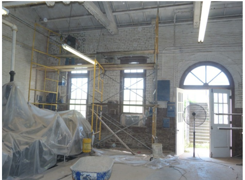
Brick mason at work repointing joints
