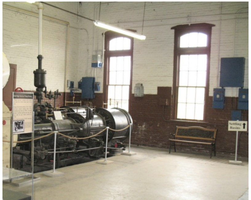
View of Old High Service Pump Room
