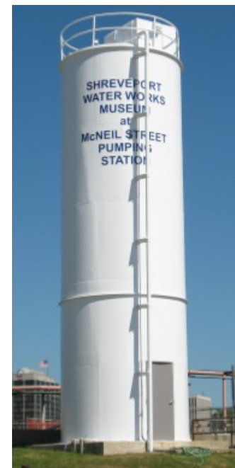
Lime tank "after"
