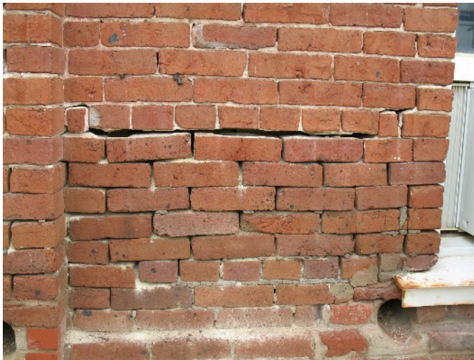
Close-up view of wall "before"
