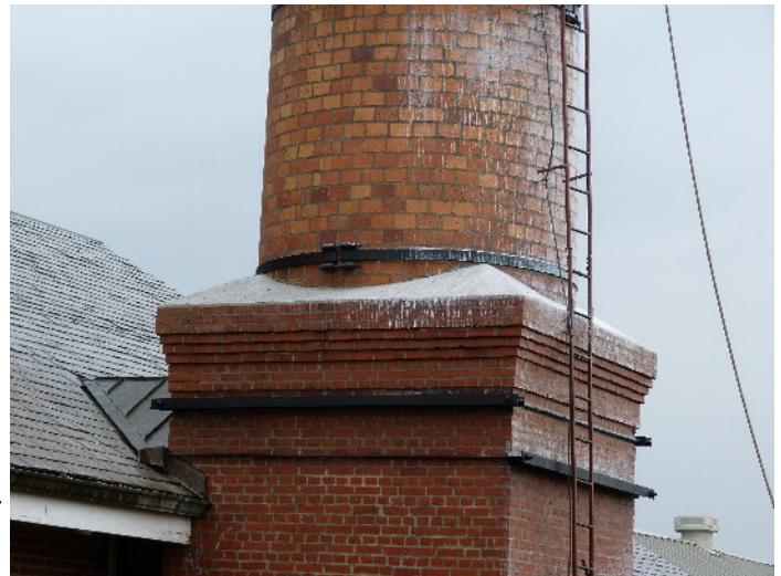
New concrete water table installed at junction of round stack and square base replacing old broken one
