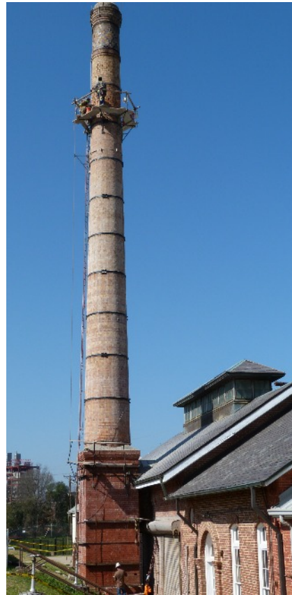
Gerard crew at work on Adolphus-Custodis chimney
