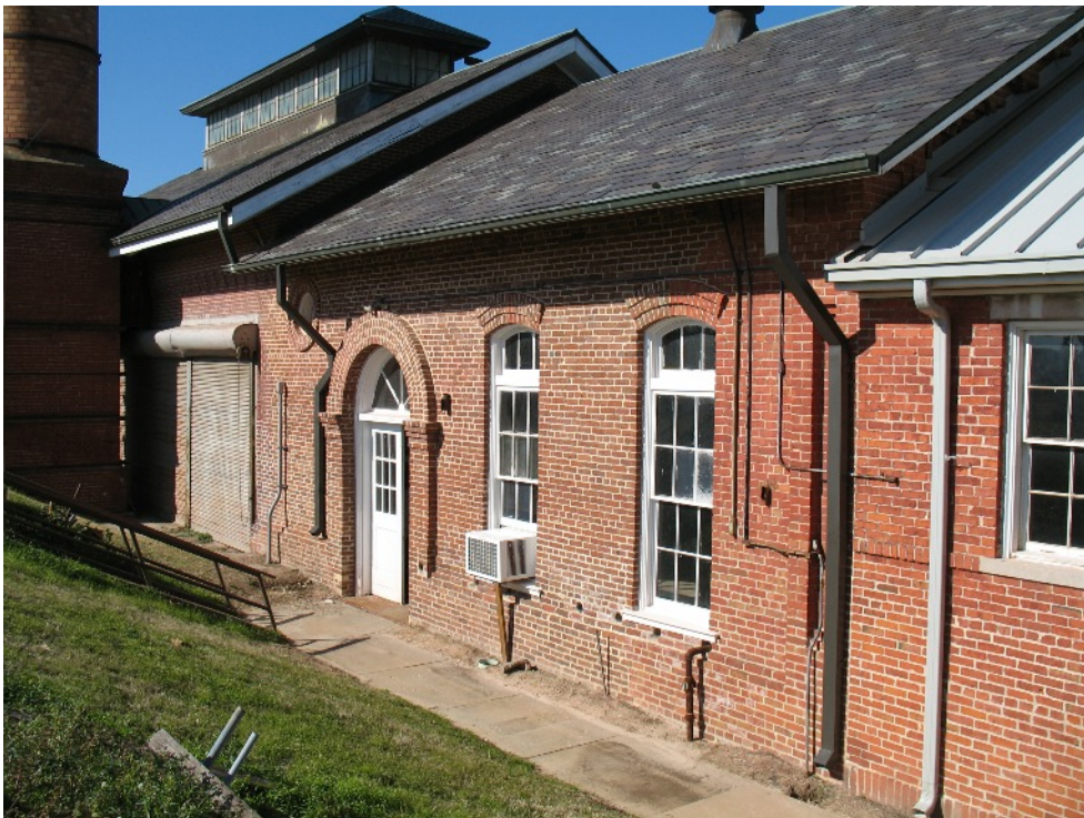
Overview of repointed south wall of pumphouse
