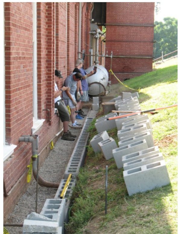
Scout crew with mostly completed retaining wall
