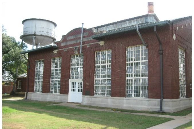
Front view of main pump room added in 1921
